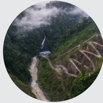
PLTA Pakkat 18 MW (North Sumatera)
